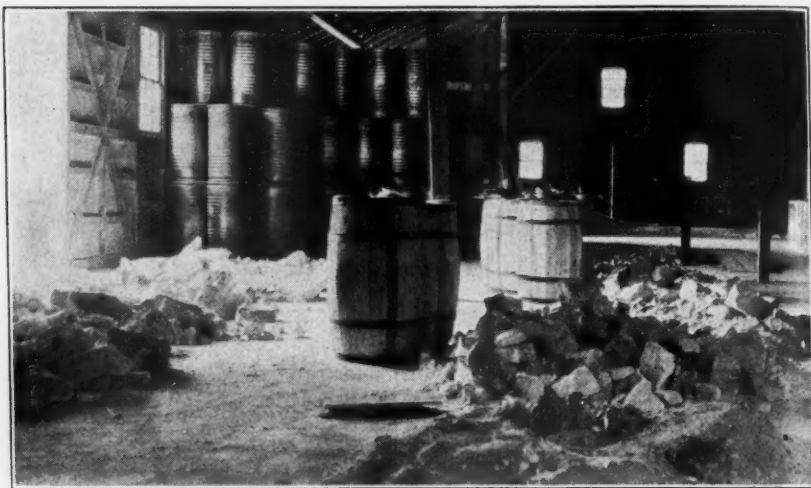
Cooling Floor, Note Wood and Steel Barrels.
